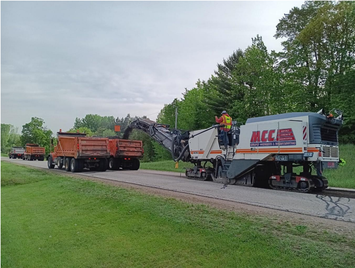
Milling on CTH BB rehabilitation project
