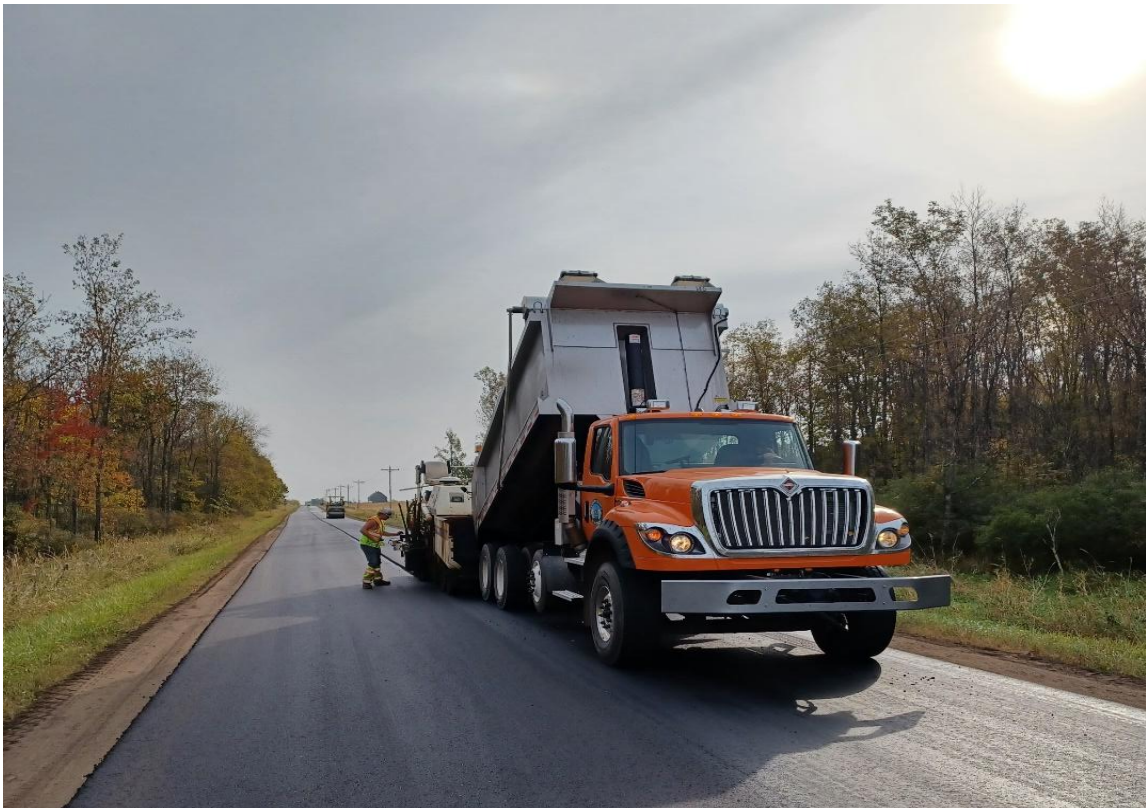
Surface paving on CTH WW rehabilitation project
